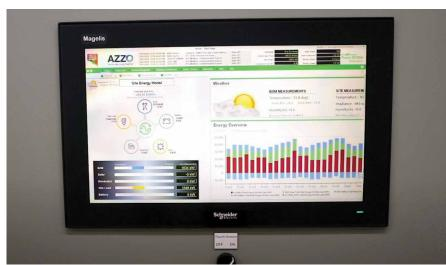
South Australian electricity spot price to protect the Market precinct from high electricity pricing and determines the optimum combination of producing energy onsite and when it is cost effective to purchase power from the grid. As a result of this combination, the total electricity charged to tenants
